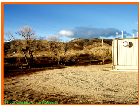
Defensible Zone Around Plant at Left Hand Canyon After Neva Fire
