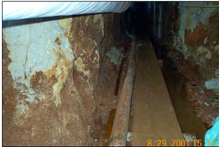
HDPE PIPE BETWEEN BULKHEAD AND STA 6+50 (2001)
