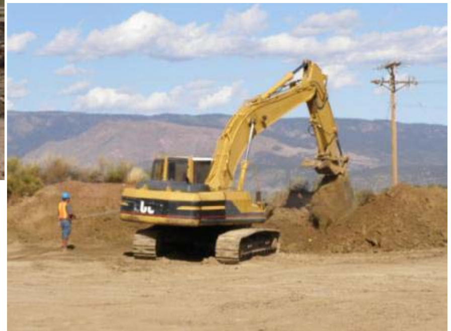
Front gate ore pad (taken 10/19/09)
