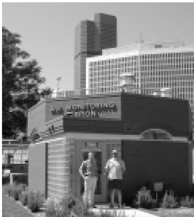
Construction of the state Air Pollution Control Division's new Denver Continuous Air Monitoring Project (CAMP) station was completed in May 2000 at 21st Street and Broadway. The previous station, a geodesic dome structure, had been in operation since 1965.
